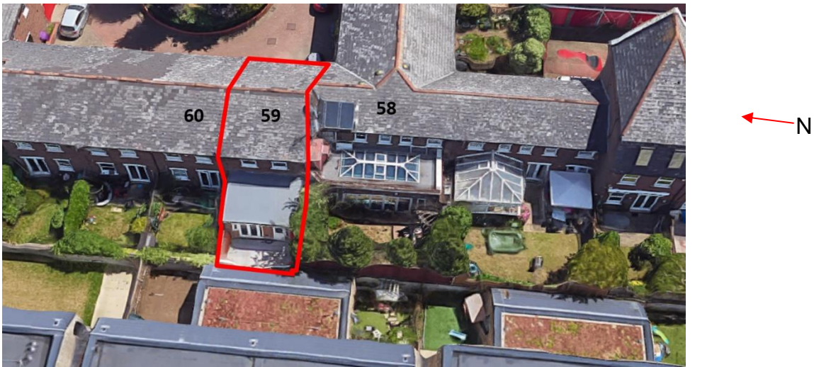
Figure 1 – Aerial photograph of the Site, with the subject and adjoining properties numbered
